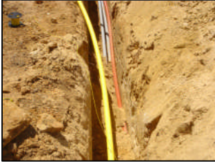
Tracer Wire Installation
