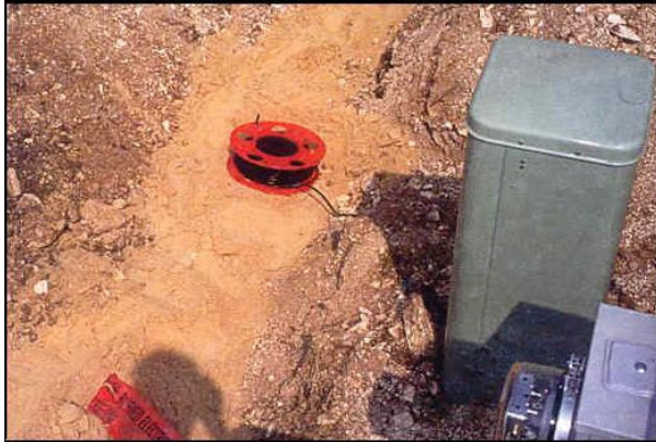
Pre-wired Locatable Service Drop
